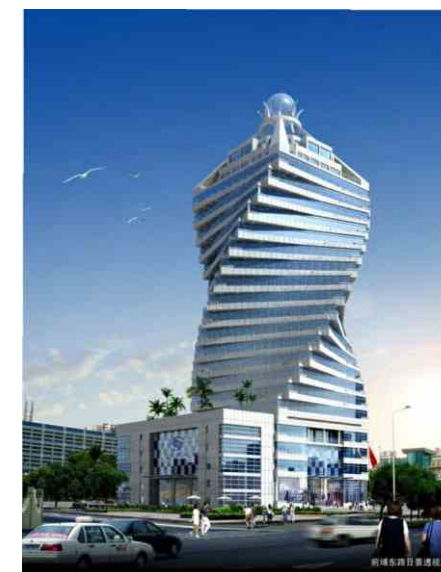
Ruihua Technology Building, Xiamen, China
