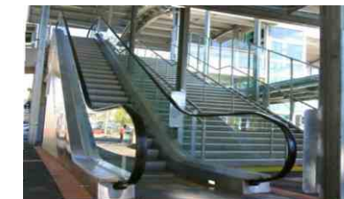
Mt Druitt Railway Station, Australia
