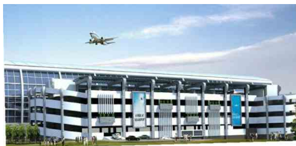
Goa Airport, India
