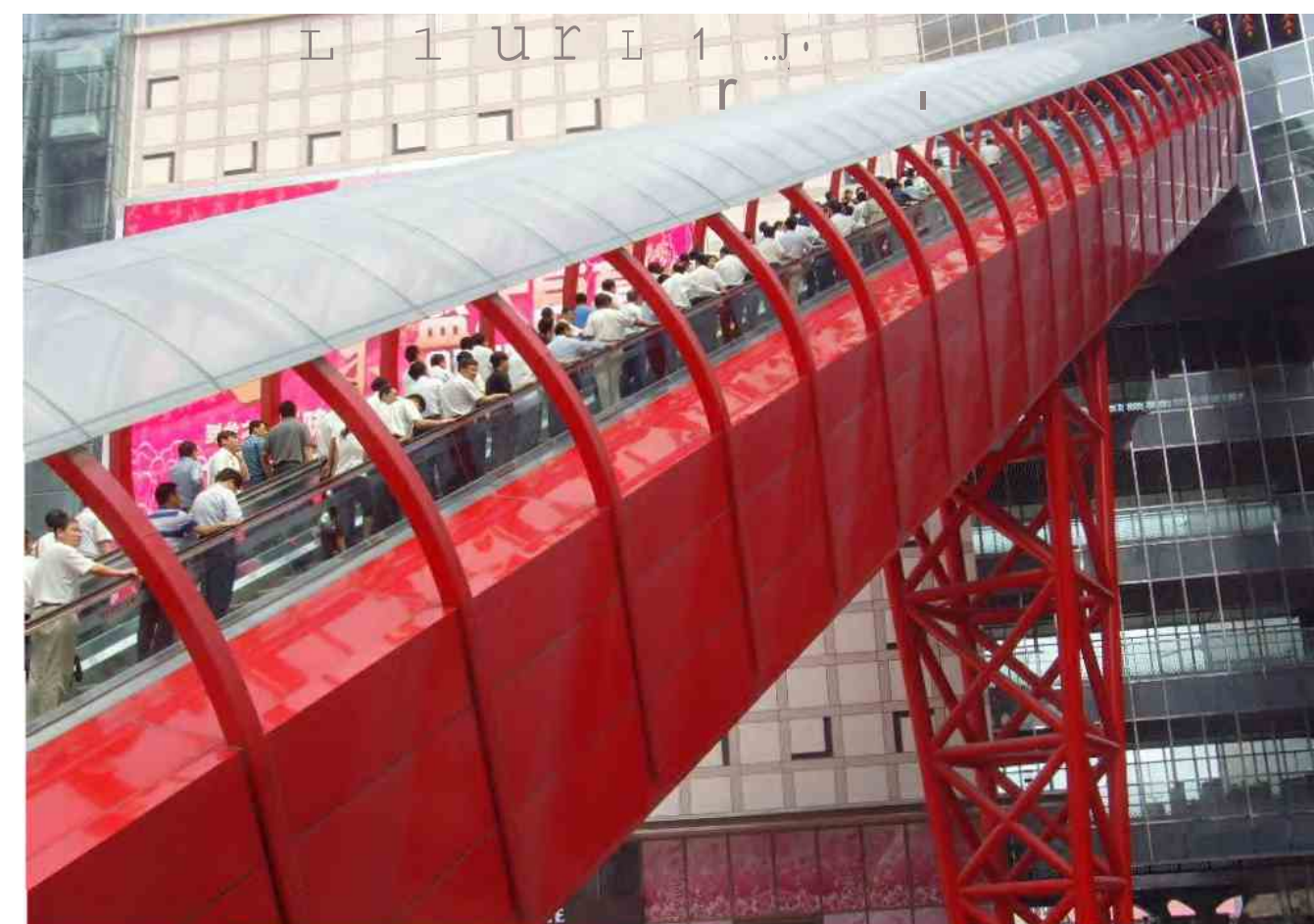
High Rise Escalator – 33.5m (2013)
